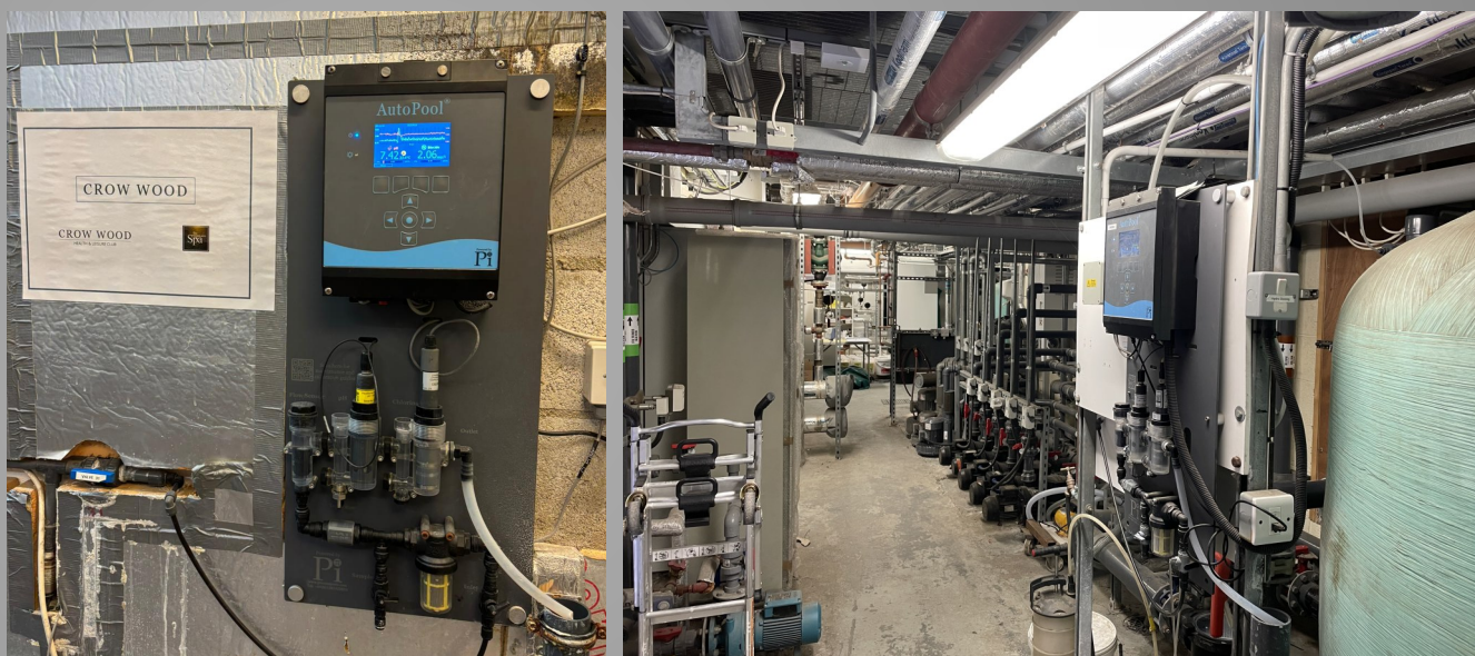
Figure 8: The AutoPool® 4.0 Chlorine mounted in the plant rooms at The Woodland Spa.
